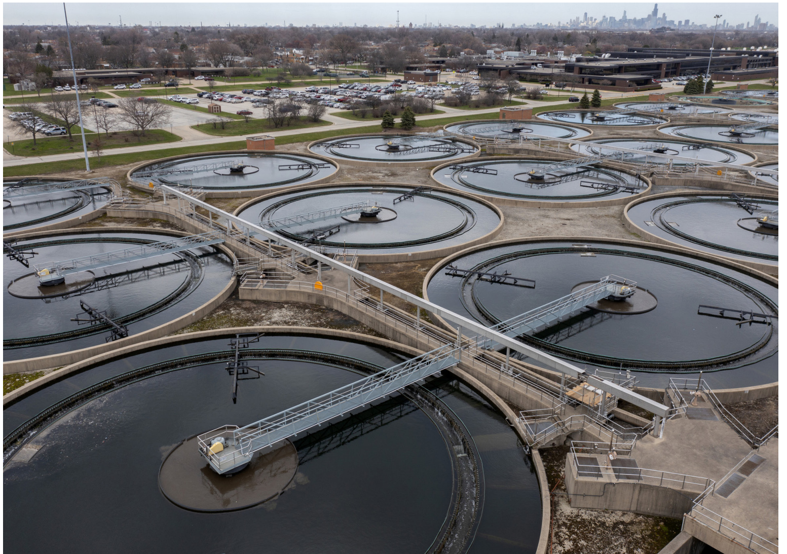
An aerial view shows the Stickney Water Reclamation Plant, operated by the Metropolitan Water Reclamation District, on April 12 in Cicero. The MWRD has been known for more than a decade that its sludge is contaminated with forever chemicals. ERIN HOOLEY/CHICAGO TRIBUNE
